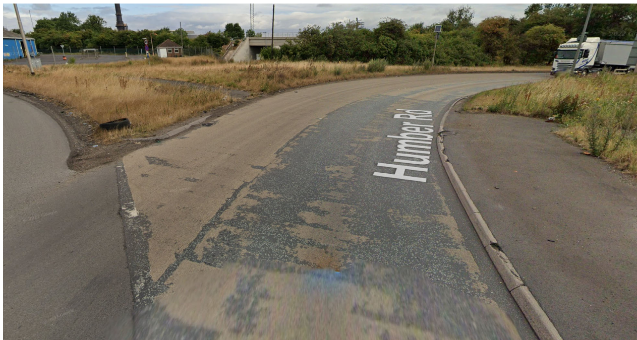
Figure 2 Existing Humber Road approach to Manby Roundabout
